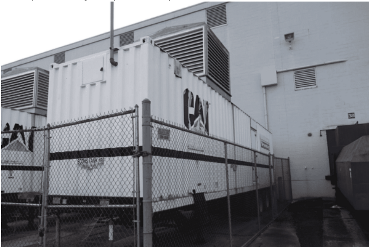
Data Center Backup Power Generators
